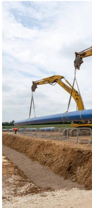
>1,000km of mains renewal
